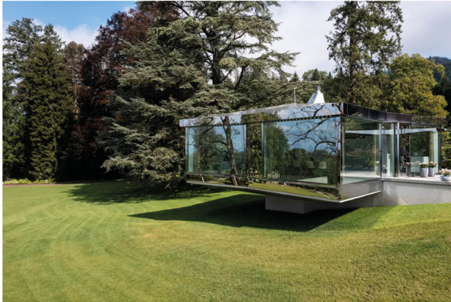
At the end of the red driveway, visitors are greeted by the newly built glass pavilion, designed by Neon Deiss Architecture, built in the form of a crystalline mirrored glass structure which provides space for dining, meetings, and events. The architectural garden has been redesigned to include a natural pool, tennis court and flower garden completed with a pergola for outdoor dining, relaxation, and enjoyment. Reto Guntli & Agi Simoes
